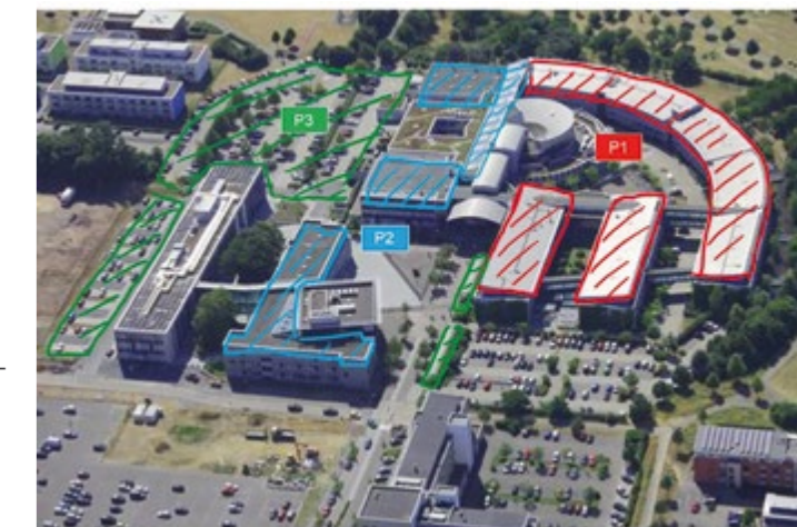
Plenty of potential: The roofs, carparks and green areas at H-BRS offer sufficient space for photovoltaic systems
